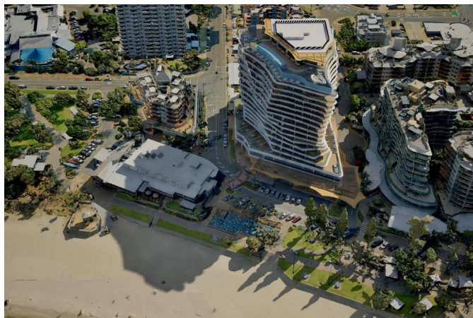
Summer solstice - Dec 21 @ 4pm (Top to bottom - approved version vs lodge version vs revised version)
