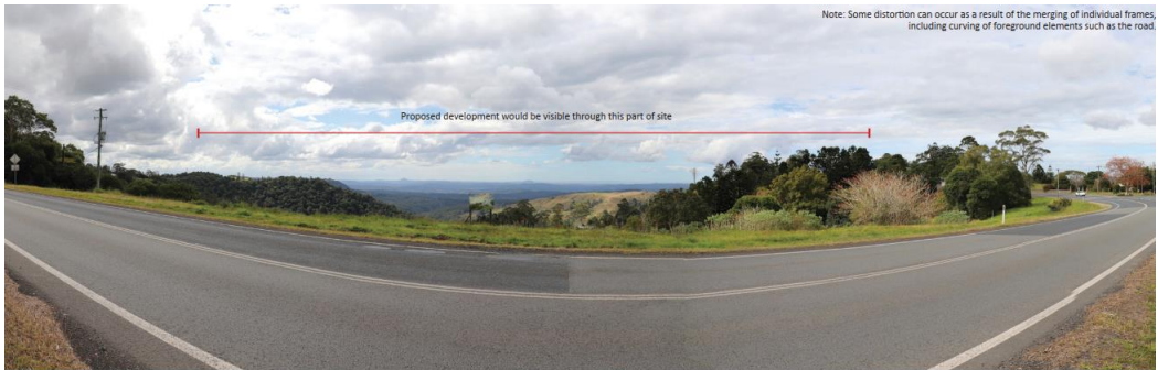
Figure 20 View of site from Landsborough Maleny Road
