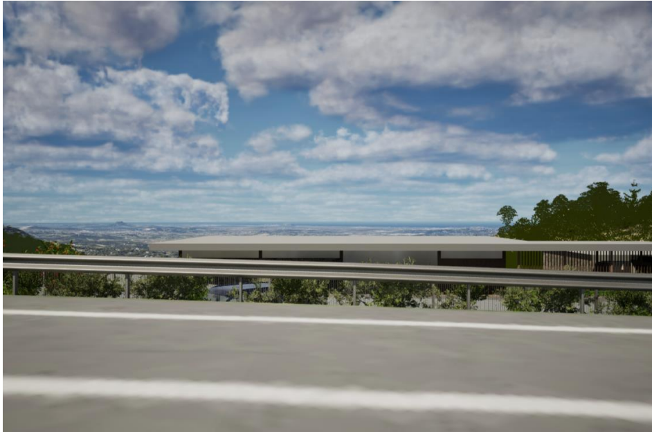
Figure 32 Council 3D model view of proposal from Landsborough Maleny Rd from Viewpoint D
