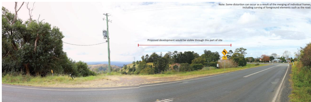
Figure 18 View of site from Landsborough Maleny Road
